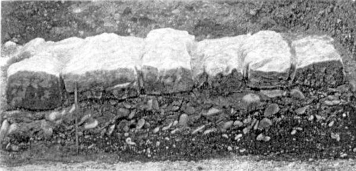
1. Foundation of the reducing wall
